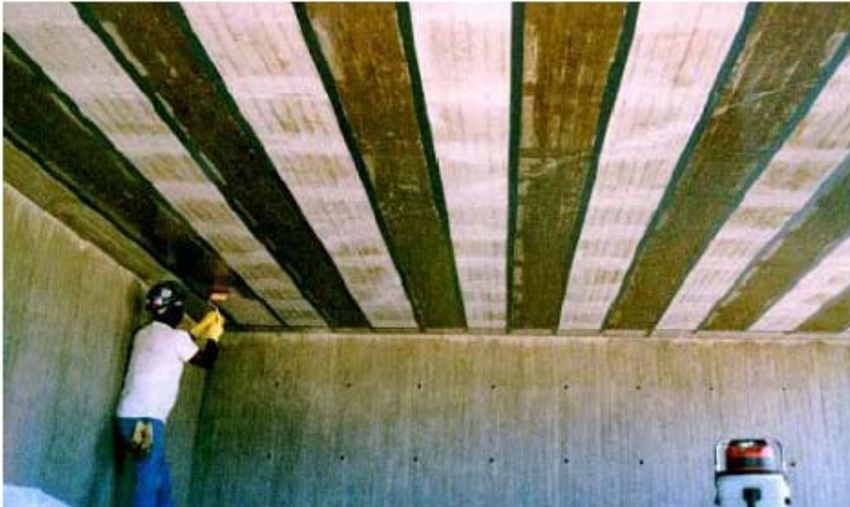
Fig. (2-8): Application of Epoxy Primer, [ISIS-EC-6, 2006].
