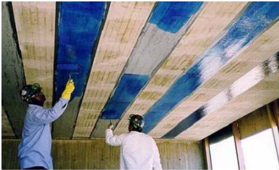
Fig. (2-10): Application of Epoxy Saturant Layer, [ISIS-EC-6, 2006].
