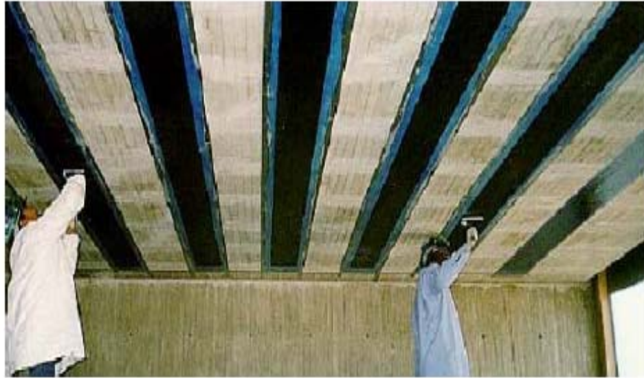
Fig. (2-11): Impregnating of CFRP Fabric with Epoxy, [ISIS-EC-6, 2006].
