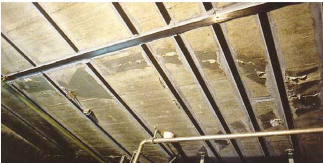
Fig. (2-4): Two-Way Flexural Strengthening of a Reinforced Concrete Slab Using Carbon FRP Strips, [ISIS-EC-4, 2004].
