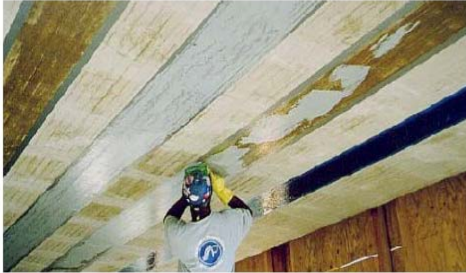
Fig. (2-9): Application of Epoxy Putty, [ISIS-EC-6, 2006].
